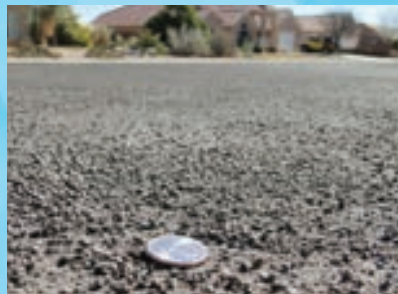
TYPE II SLURRY (Approx. 6 months after Type II Slurry was installed)
