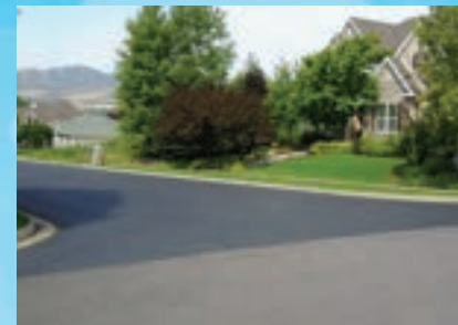
HA5 HIGH DENSITY MINERAL BOND (Approx. 3 years after HA5 was installed)
